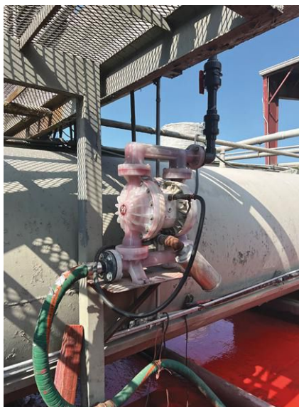
IMAGE 2: Fire retardant treatment for wood using a 2-inch AODD pump
