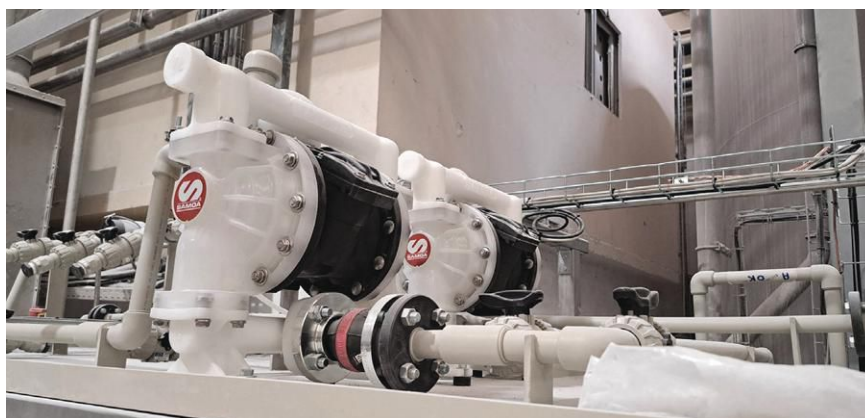
IMAGE 1: Biocide paint applied using a 1-inch AODD pump (Images courtesy of SAMOA Industrial)
